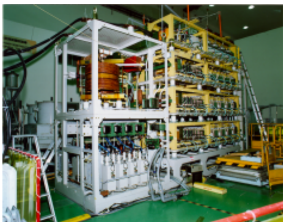
Fig. 2 One of the four stages (1/4 valve) of a 53MVA converter.
