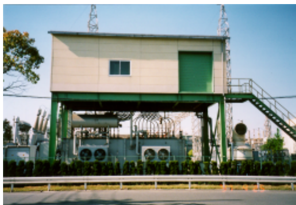
Fig. 5 A 20MVA Compact STATCOM installation.
