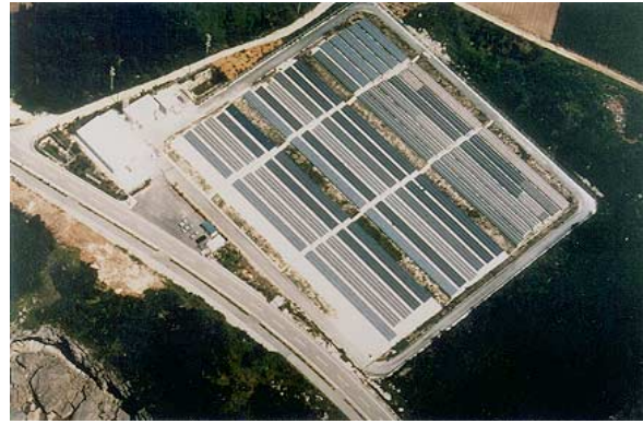
Fig. 1 An aerial view of the pilot plant.
