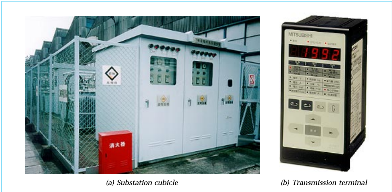
Fig. 2 B/MRU1 transmission terminal built into a substation cubicle.
